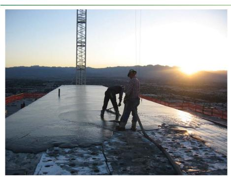
MEARLCRETE™ is a traditional protein based foam liquid concentrate. Lightweight insulating concrete (LWIC) using protein foaming agents has been around since the 1940's with a long track record of success in the roofing industry.
