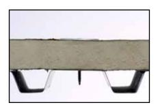
**SIDE VIEW** Correctly installed plate/fastener. Minimum 3/4" penetration through roof deck.
