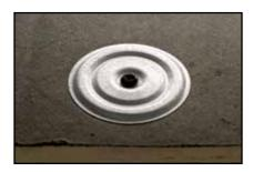
**TOP VIEW** Correctly installed plate/fastener.
