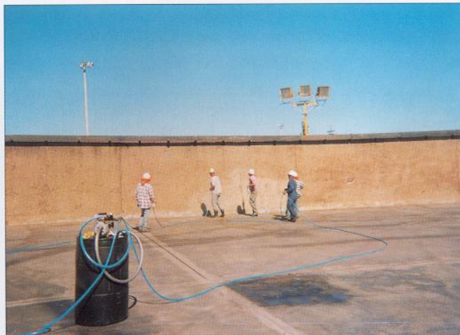
FIGURE 38 - RADCON #7 APPLICATION
