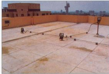
FIGURE 24 - ROOFTOP WITH INSULATION AND TOPPING
