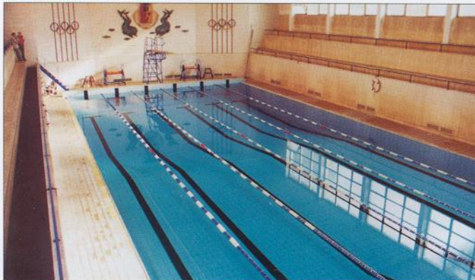
FIGURE 30 - SWIMMING POOL RE-FILLED AFTER SUCCESSFUL REPAIRS
