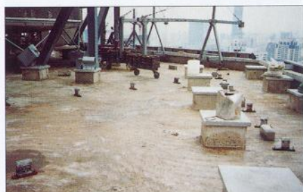
FIGURE 15 - RADCON #7 TREATED
