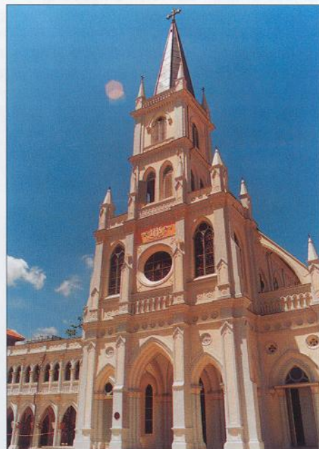
FIGURE 20 - 140 YEAR OLD CHURCH RESTORED
