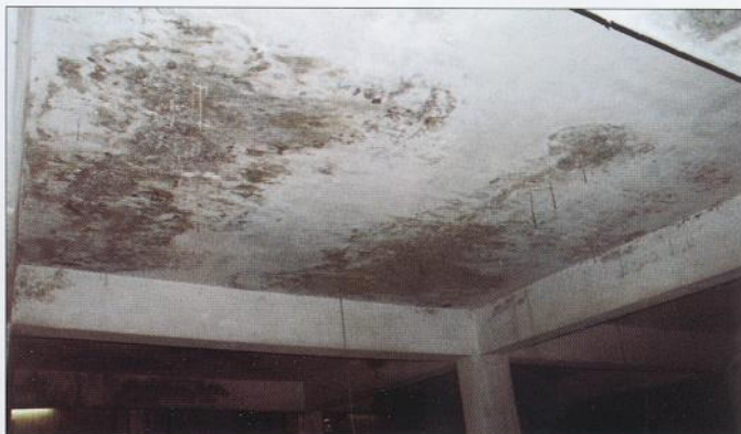
FIGURE 31 - SOFFIT WITH 300MM CALCIUM STALACTITES
