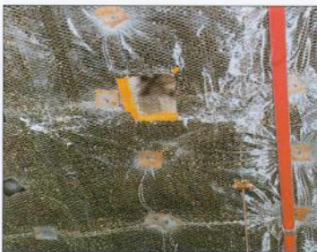
FIGURE 40 - INSULATION ON THE SOFFIT
