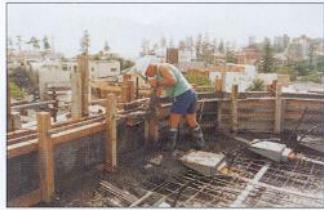
FIGURE 10 - CAST IN-SITU PARAPETS
