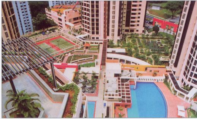
FIGURE 25 - LOOKING DOWN ONTO SUSPENDED PODIUM DECK
