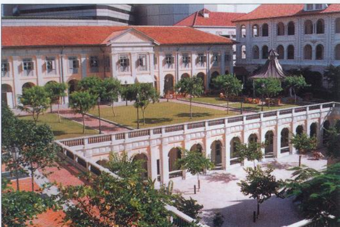
FIGURE 19 - THE SUNKEN COURT YARD, C.H.I.J.M.E.S.
