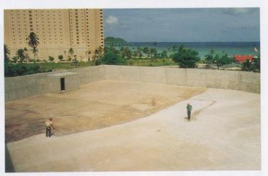
becomes touch dry again. This watering must be carried out within 6 hours of product application. Step 4 begins the waterproofing action of Radcon #7 as the product reacts with the water and free lime to form a glass hard water repellant gel in the pores, cracks and capillaries deep into the concrete. The watering procedure is repeated the next day and then on the third day the area is ponded to verify that a complete seal has been achieved.
