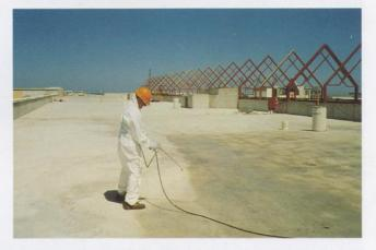
Surfacing and the applicator can be seen in the bottom photo using a motorised spray unit that enables Radcon #7 to be applied at 600 to 800 square metres per hour.
